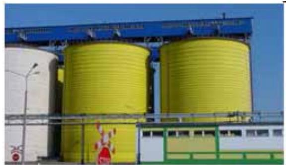
d. Silos strengthened with external prestressing in Brej (PL) (Freyssinet, 2009)
